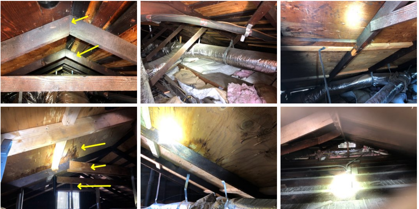
Damage at framing- soft spots noted when walking roof- in need of repair
