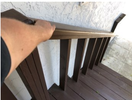
Loose railing/not grippable.
