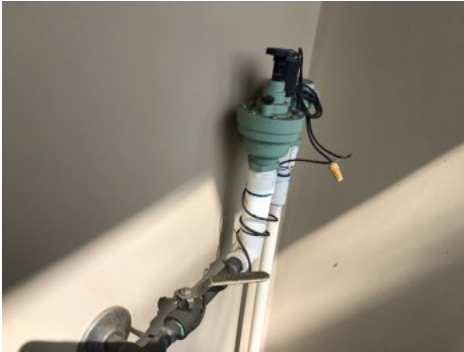
Sprinkler valve- drip system at patio
