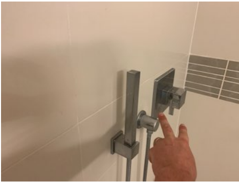
Defective valve- not working
