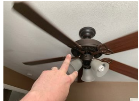
Light not working- pull cords missing
