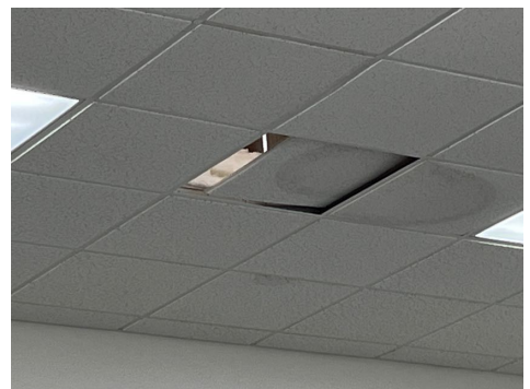
Loose- storage warehouse
