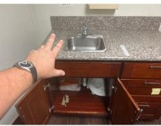
Sink not working disconnect drain line- rear office 4
