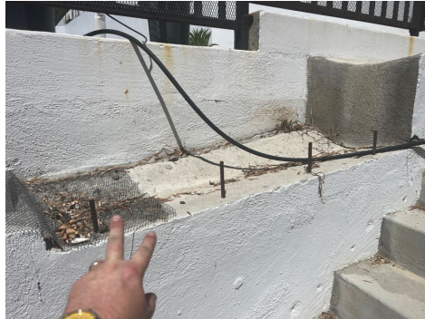
Exposed rebar
