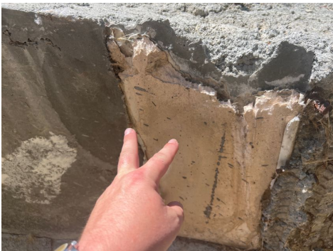
Exposed cement board/backer board.
