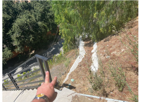
missing railing
