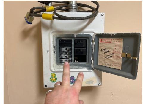
Missing screw/unprotected opening - storage room
