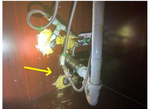
Oxidation/corrosion- rear office/sink area
